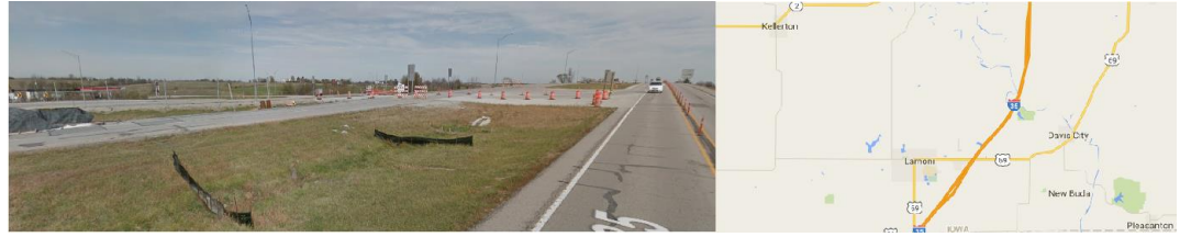
Fig 21: Work zone 5.1 in October 2015, very wide median; Source: Google Maps
